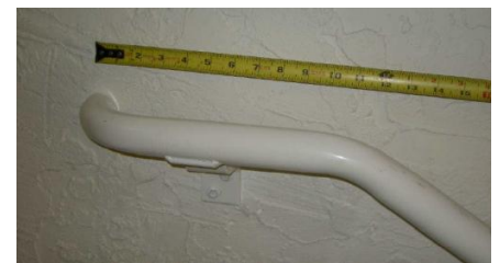
Example of compliant handrail at top riser
